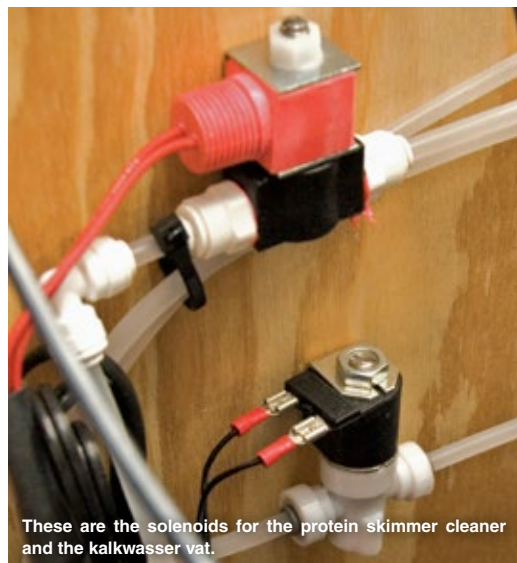
These are the solenoids for the inlet, wastewater, purge, RO/DI vat, and saltwater mixing vat.
