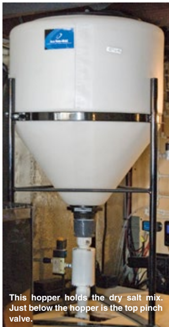
A compressed air source is used to open and close the pneumatic pinch valves.
